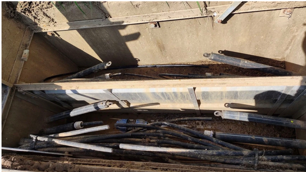
Exhibit 12: Fiber optic cables cut in several locations in France prompting an criminal investigation (Source: CYBERSCOOP)
