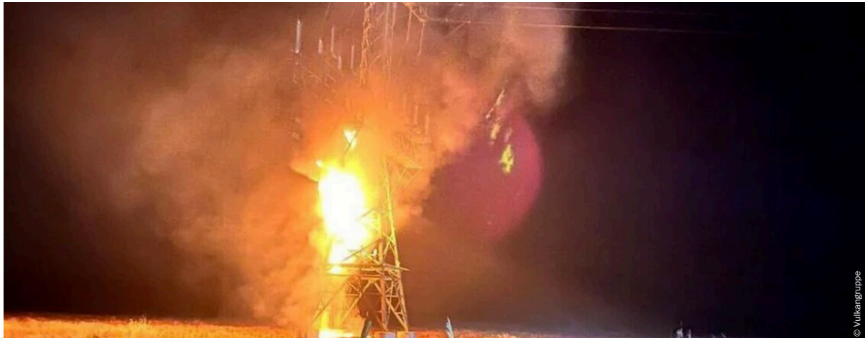
Exhibit 13: Arson attack on the power supply of the TESLA factory in Brandenburg/Germany (source: Handelsblatt, 6 March 2024)
