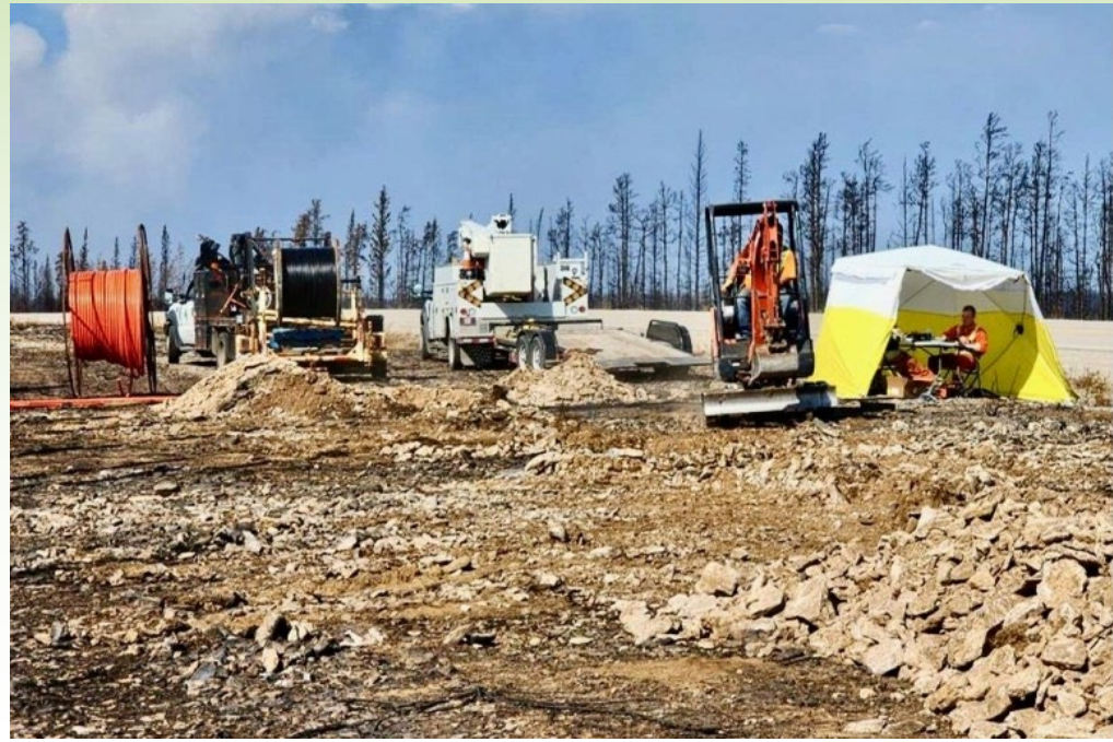
Repairing fiber after remote wildfire, 2023
